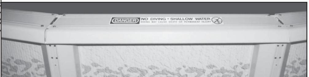
Place ledges over the wall with each end resting on a top plate. Using the above chart as a guide align the set of holes in the top plate as shown in the above drawing for your size pool with the holes in the ledge and insert the No.12x1/2" Sheet Metal Screw through the ledge and into the top plate. The actual screw holes that are used does not affect the integrity of the pool. You may use the set of holes that line up best!
