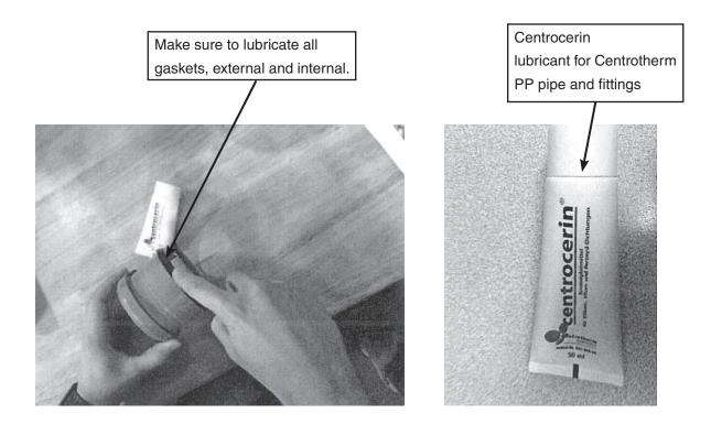
The PVC to PP adapter should then be installed into the PVC couplings on the inlet air and exhaust vent installed on the unit. The sealing gasket will require some type of lubricant to make it easier to install the adapter.
