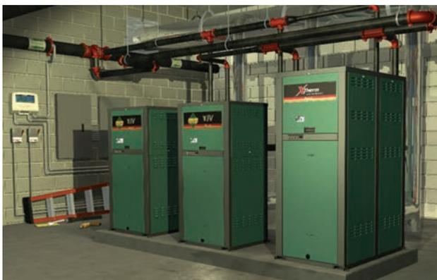
Hybrid system using 2-MVB's and 1-XTherm
